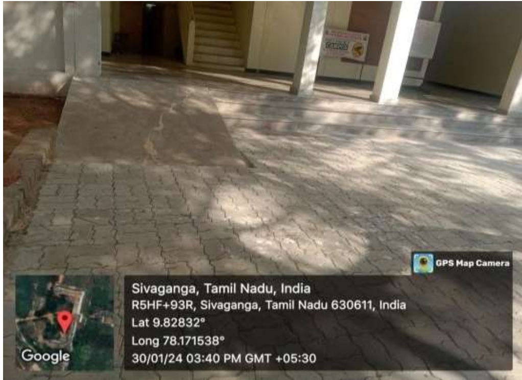
Ramp at the Ground floor of Main Building for differently abled persons
